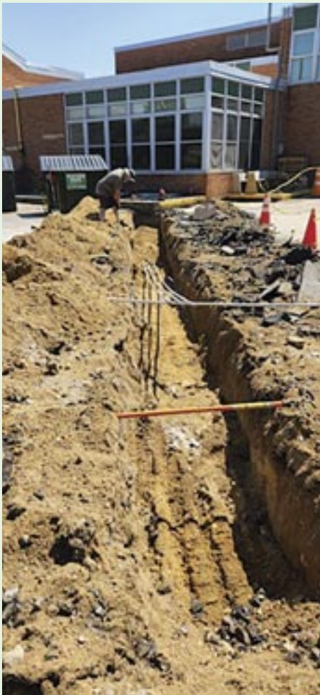
Sean Dimperio from Brentwood schools drilling through 14 inch concrete to run the electric, for a new sign and then backfilling the lines at South Middle School.
